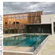
Groupeement (Eiffage Construction Equipements, Coste Architecture, Patrick Tuail, Clévia) © C. Lauté - SQY
