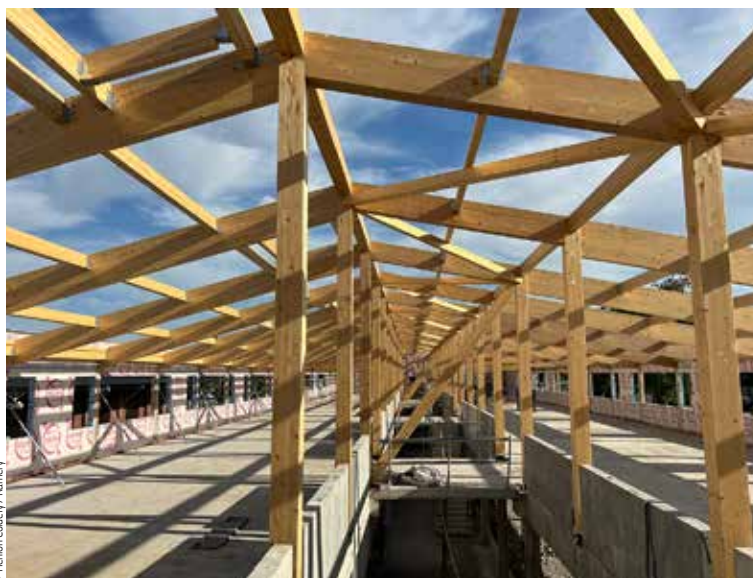
Charpente bois, collège Robert Badinter, Cambrai
