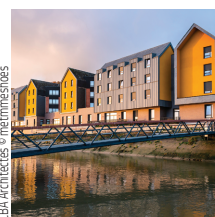
CBA Architectes © meimesmes
