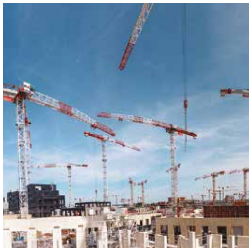
© LeoCrouzille © Eiffage Construction
